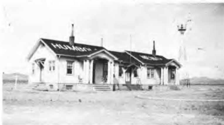
HUMBOLDT, NEVADA Keeper and Weather Station Intermediate Landing Field.
